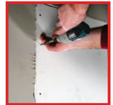
Gypsum board application
