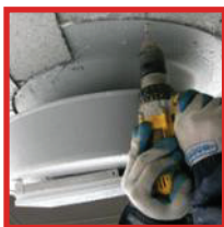
Fixing Air handling unit & ventilators
